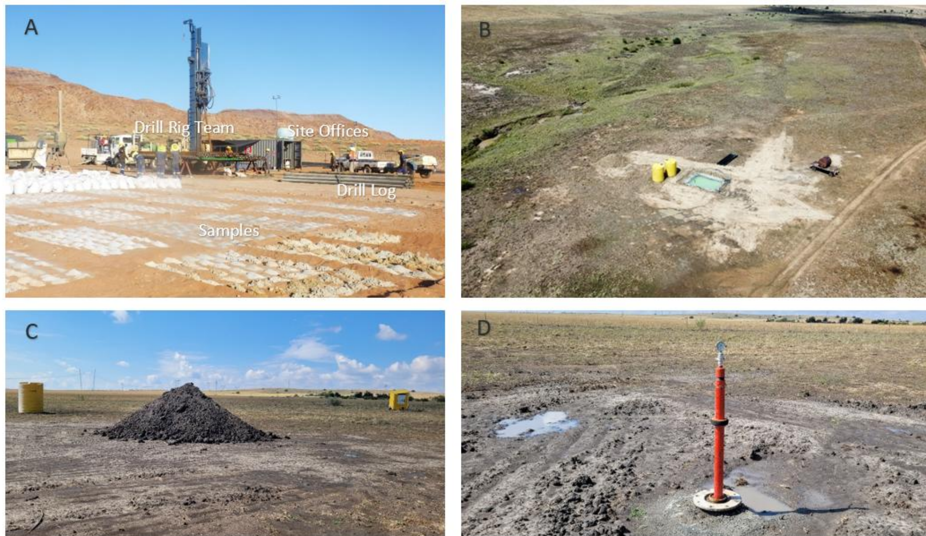
Figure 8: Exploration drilling and potential impacts. (A) Showing the drilling process and associated infrastructure, (B) Showing the drill pad footprint at one of the active D3 Energy drilling sites, (C) Showing some of impacts associated with drilling activities including controlled vegetation clearance and topsoil stockpiles and (D) Showing the final borehole, steel cased and have cemented to prevent leaks.
